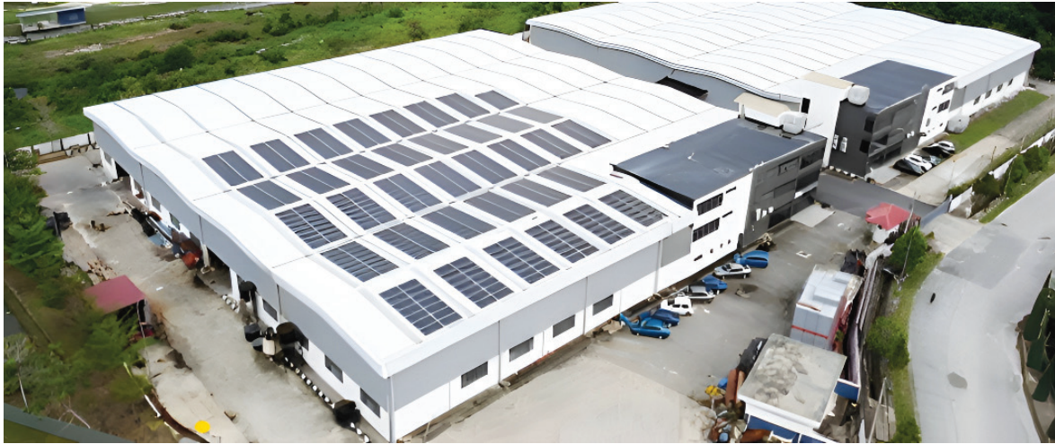
Solar PV Installation at Fibromat Rasa Facility
