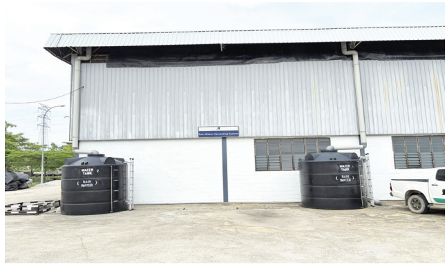
Rainwater tank for general purposes
